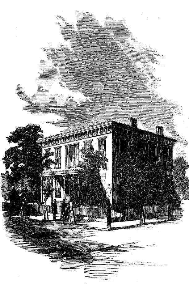
THE WHITE HOUSE AT MONTGOMERY—RENT $5000 A YEAR.
