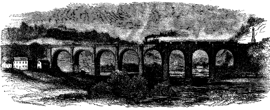
THE WASHINGTON JUNCTION VIADUCT, COMMANDED BY THE WINANS GUN AND FEDERAL ARTILLERY.
